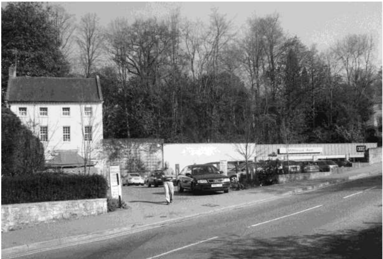
The site of the later 'Bennet's Mill', left to Scarborough Chapman by the will of his aunt Jane Swanton. The road on the right runs through the old mill ground.
